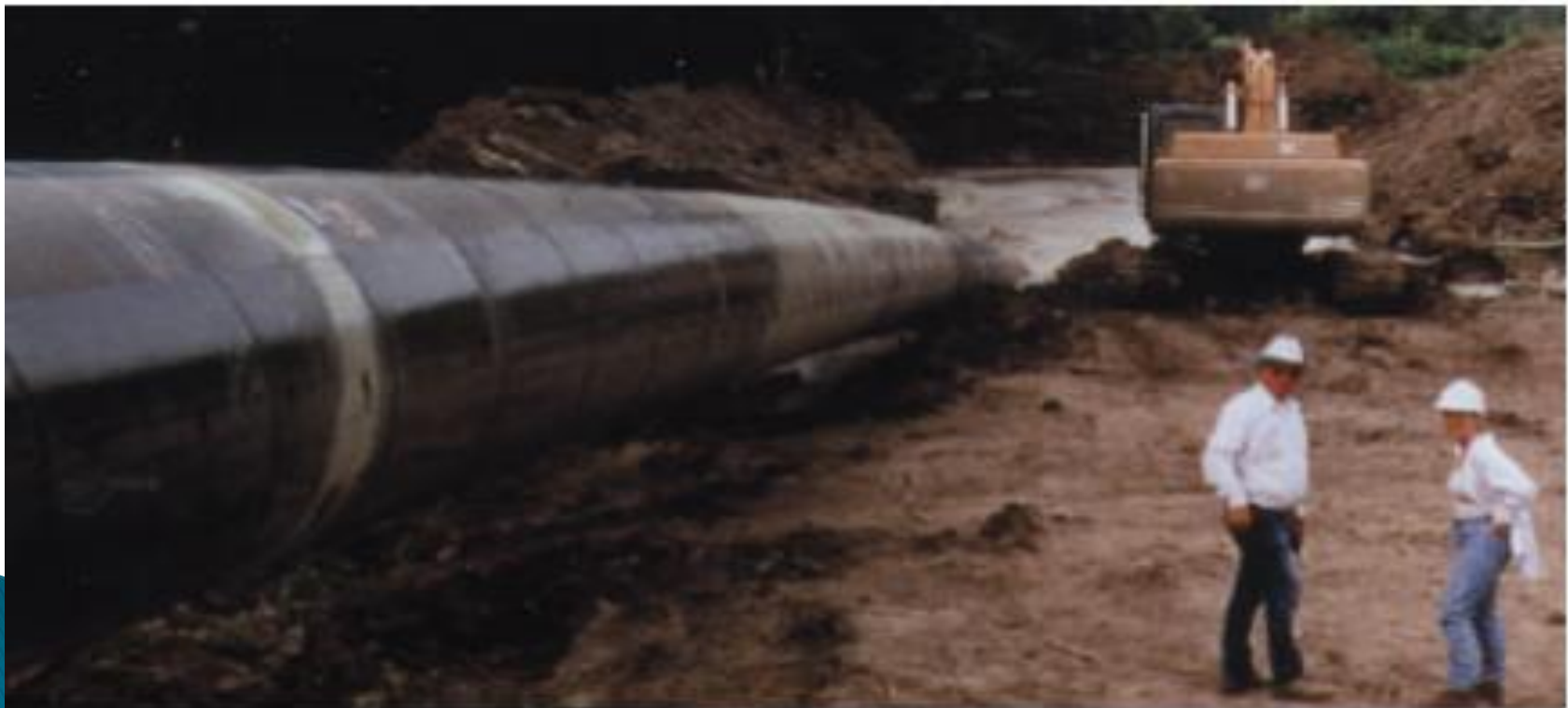
Figure 4. Entrance of 48 in. pipe at Guadalupe River Crossing.
