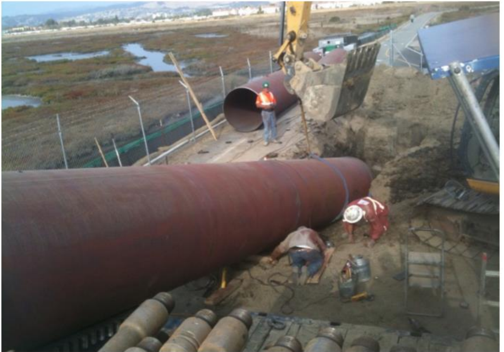
Figure 5. Conductor Casing Being Installed at Entry Point
