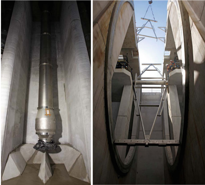
Fig. 2.13 SDP intake pump/fine screen during installation
