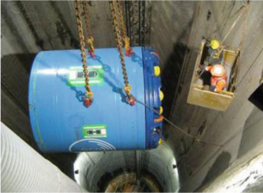
Fig. 3.12 Lowering of tunnel boring machine into the riser shaft connecting the SWRO plant to the tunnel
