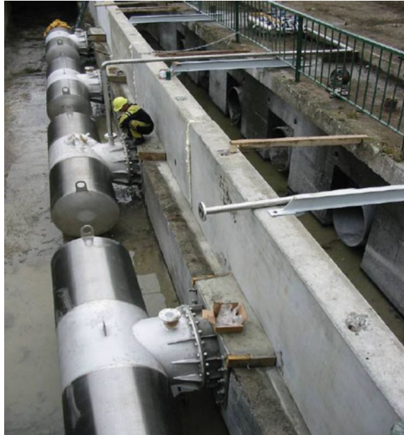
Fig. 5.1 Passive screen intake along a seawall or channel edge (Courtesy of Gap Technology Limited)
