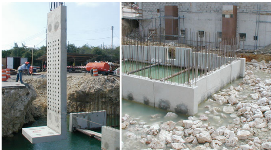
Fig. 1.5 Onshore karst pit intake in Curaçao
