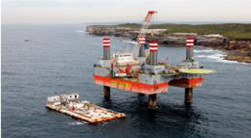
Fig. 3.5 Sydney coastline showing the intake riser site with a jack-up drilling and grouting barge
