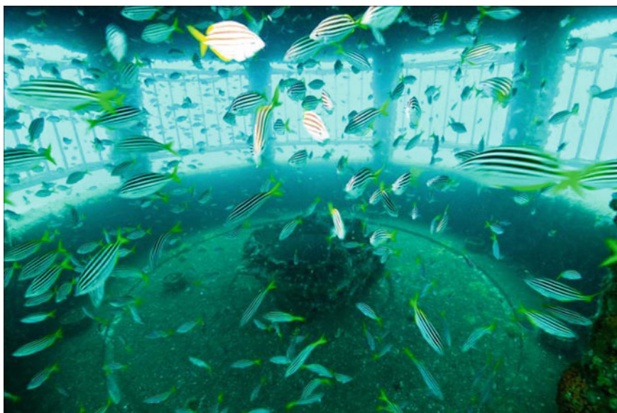
Fig. 3.9 Interior view of the velocity cap intake during operation of the Sydney SWRO plant
