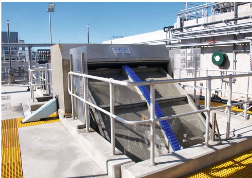
Fig. 1.2 Drum screen (From Pankratz 2007)
