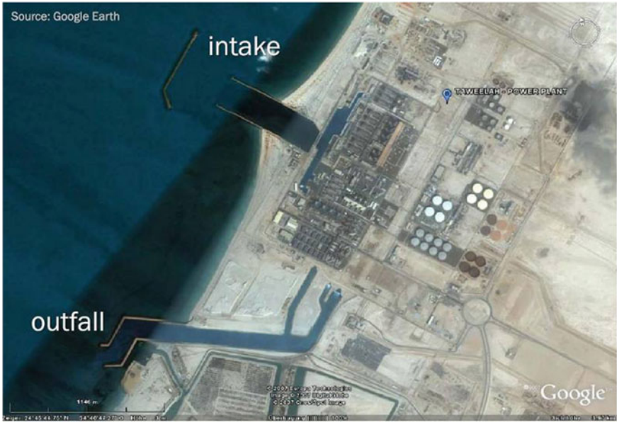
Fig. 18.6 Taweelah MSF plant, Arabian Gulf, 1.12 mio m 3 /d, positively buoyant discharge (Source Google Earth)
