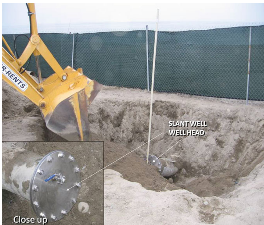
Fig. 13.5 Wellhead burial 1.5 m below land surface
