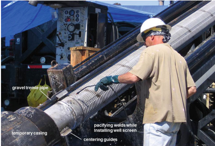
Fig. 13.20 Installing the casing and screen
