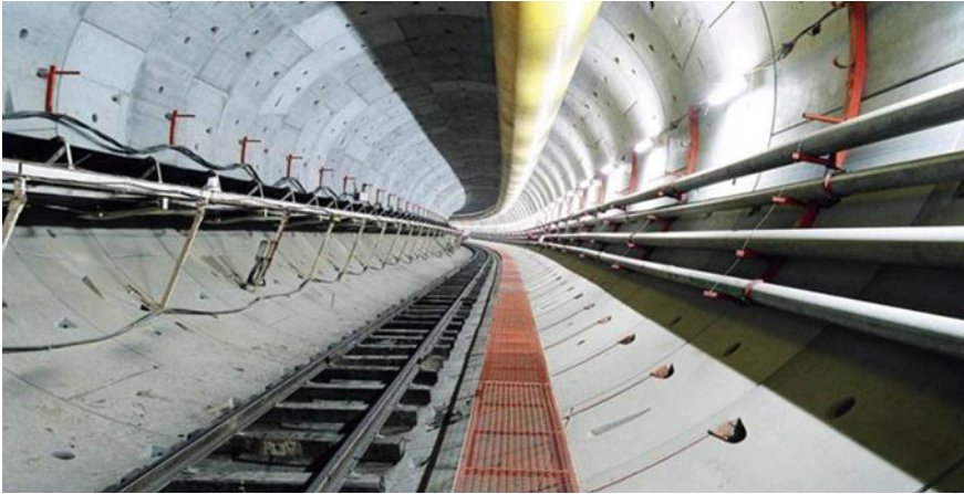
Fig. 3.3 Sydney SWRO plant intake tunnel
