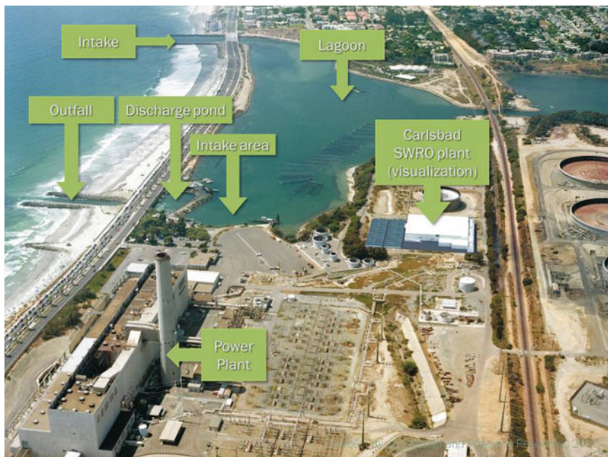
Fig. 18.4 Carlsbad RO plant, USA, positively/negatively buoyant discharge (Source Poseidon Resources)
