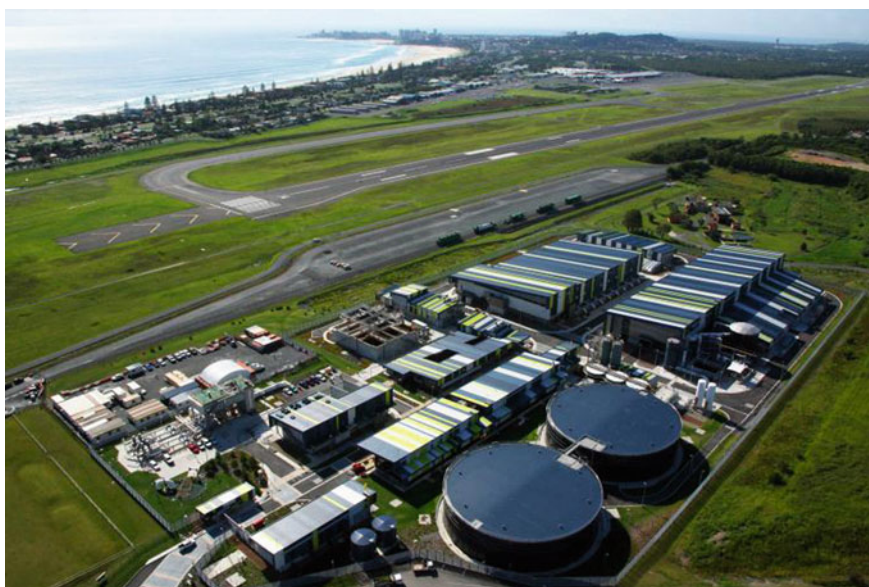
Fig. 3.10 Aerial view of the Gold Coast SWRO plant
