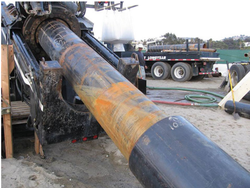
Fig. 13.21 Removal of Temporary Casing
