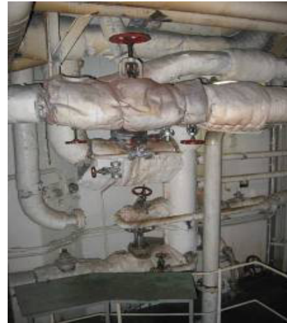
Figure 1: Typical use of asbestos as lagging on pipelines
