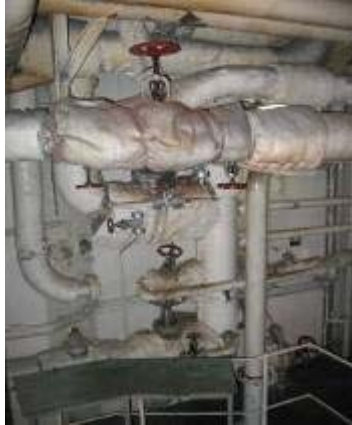
Asbestos lagging on piping and asbestos gaskets at e.g. hatches
