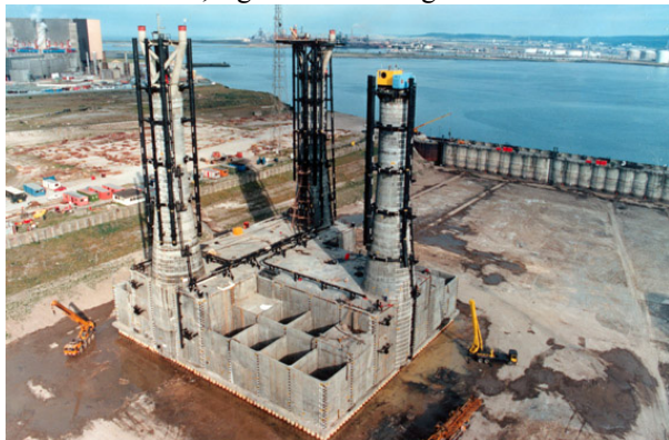
Figure 3: TERC Dry Dock – Construction of Ravenspurn GBS.
