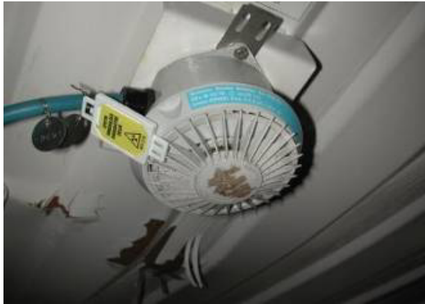
Figure 3: Typical ionising smoke detector with a radioactive source
