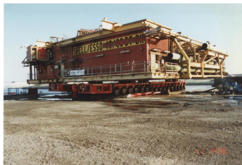
Figure 2: Load in of a 1,644tonne topside module from a barge (1996)
