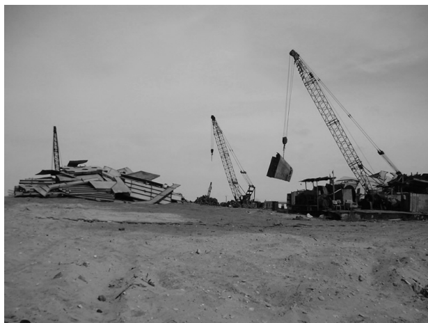
Figure 4: Panels transfer from Inter-tidal to cutting area.
