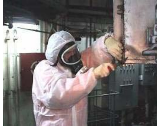
Asbestos lagging on piping and asbestos gaskets at e.g. hatches
