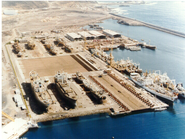
Figure 4: Dual Level System at Astican, Las Palmas
