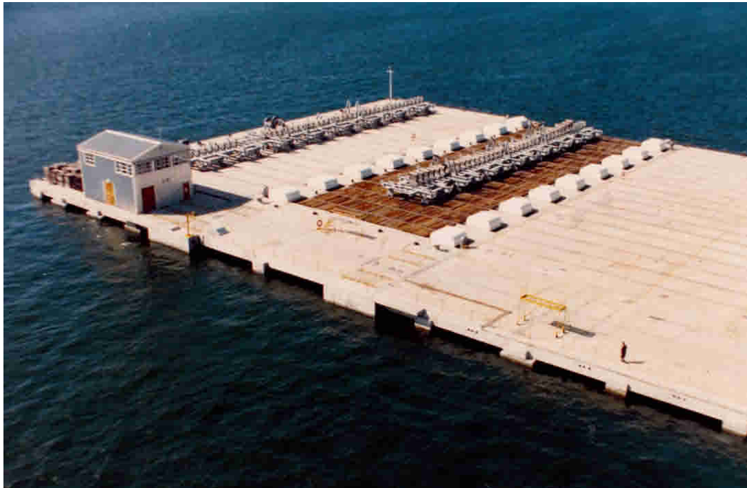
Side transfer both sides in Durban
