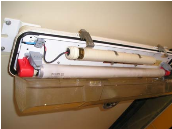
Fluorescent light tubes may contain mercury
