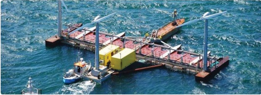
Fig. 6.1 Poseidon, an example of hybrid platforms combining wave- and wind-energy devices. (Courtesy of Sam Churchill (Churchill 2011). Original content is released under the CC-BY-SA license)
