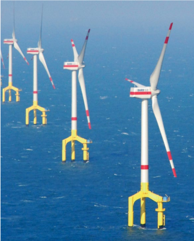
Fig. 3.10 The Bard 5.0-MW turbines supported by tripile structures at 40-m water depth at the offshore plant “Bard Offshore 1.” (commons.wikimedia.org 2013. This file is licensed under the Creative Commons Attribution-Share Alike 3.0 Unported license)
