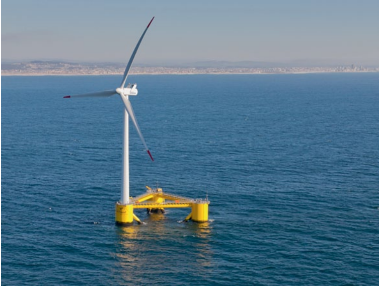
Fig. 4.4 WindFloat, a semisubmersible type floating offshore wind turbine foundation operating at the rated capacity (2 MW) approximately 5 km offshore of Agucadoura, Portugal. (Source: commons.wikimedia.org (Untrakdrover 2012); this file is licensed under the Creative Commons Attribution 3.0 Unported license)
