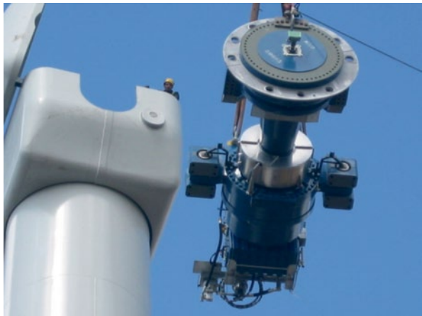
Fig. 2.7 Main shaft. (Courtesy of geograph.org.uk (Anderson, Gearbox, Rotor Shaft and Disk Brake Assembly, 2008a). © Copyright Paul Anderson and licensed for reuse under this Creative Commons Licence)
