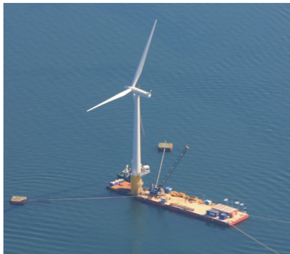
Fig. 4.3 Hywind, spar-type wind turbine. (Courtesy of Vines 2009; this file is licensed under the Creative Commons Attribution 3.0 Unported license)
