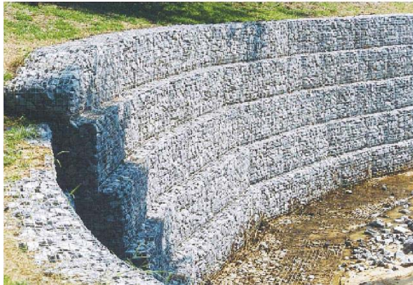
Figure 8-11. Typical gabion installation
