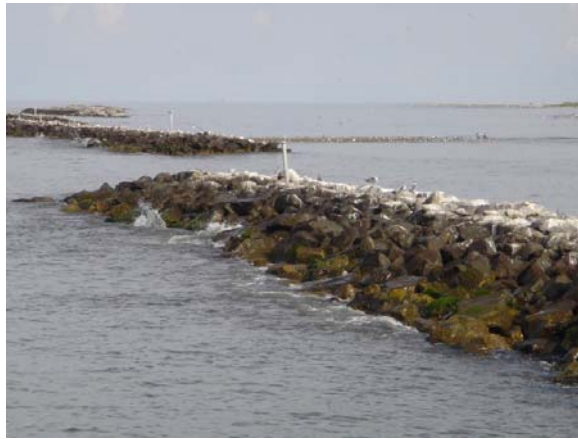
Figure 8-7. Examples of small breakwaters
